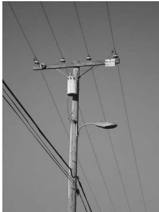
Figure 5-13. Transformer connections.
