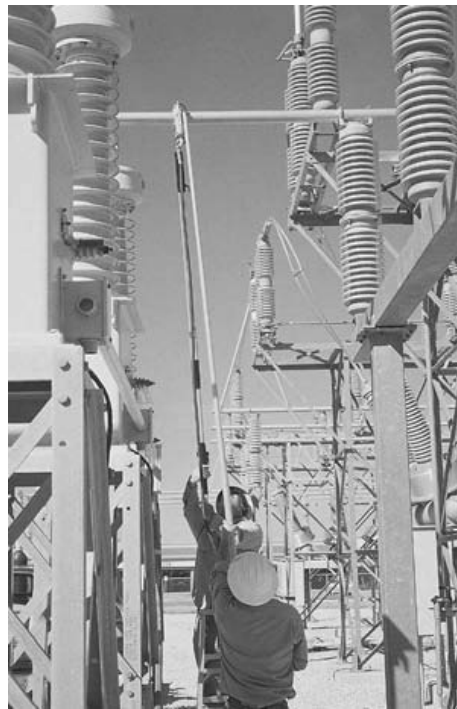
Figure 10-8. Live maintenance on transmission lines.
