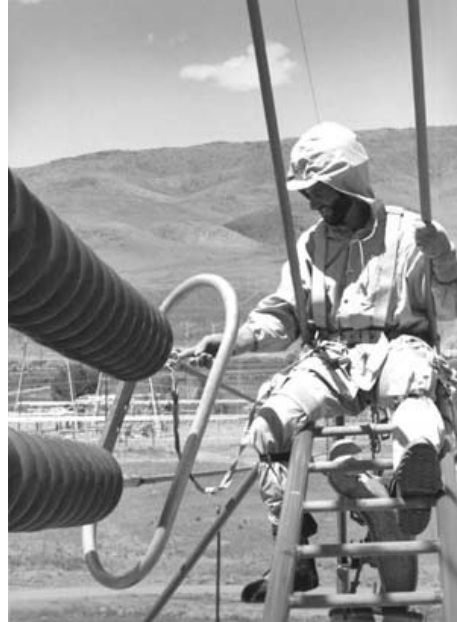
Figure 10-9. Bare-hand, live-line maintenance.
