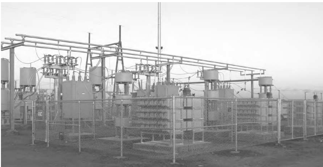
Figure 4-42. Static VAR compensator. Courtesy of Jeff Selman.
