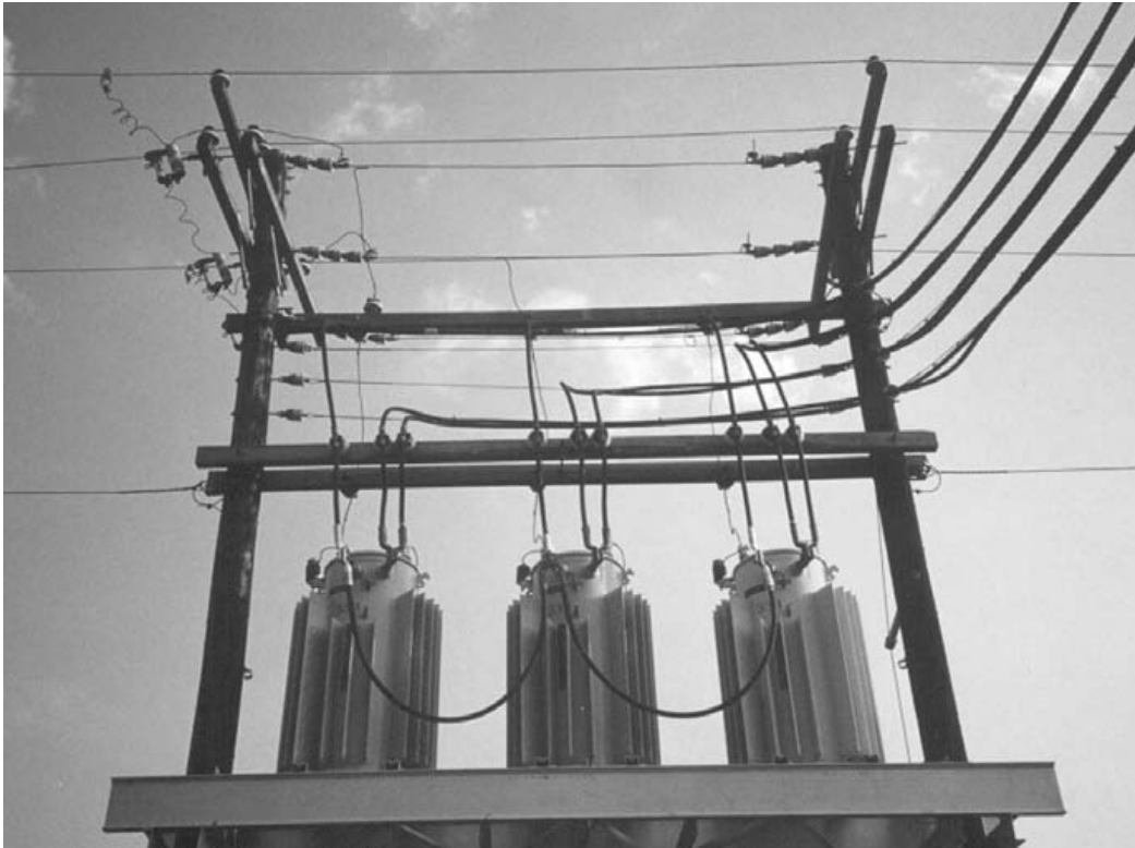
Figure 4-3. Transformer bank.
