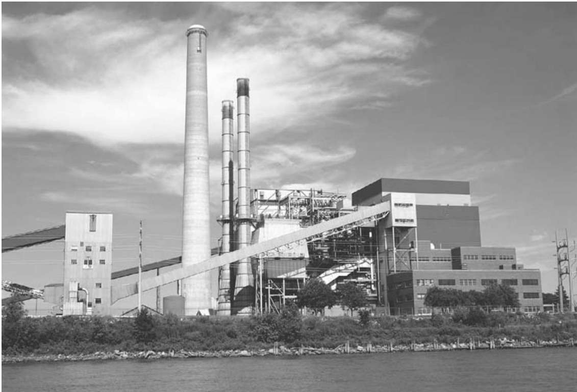
Figure 2-11. Coal power plant. Source: Fotosearch.
