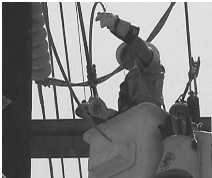
Figure 10-11. Live maintenance distribution. Courtesy of Alliant Energy.
