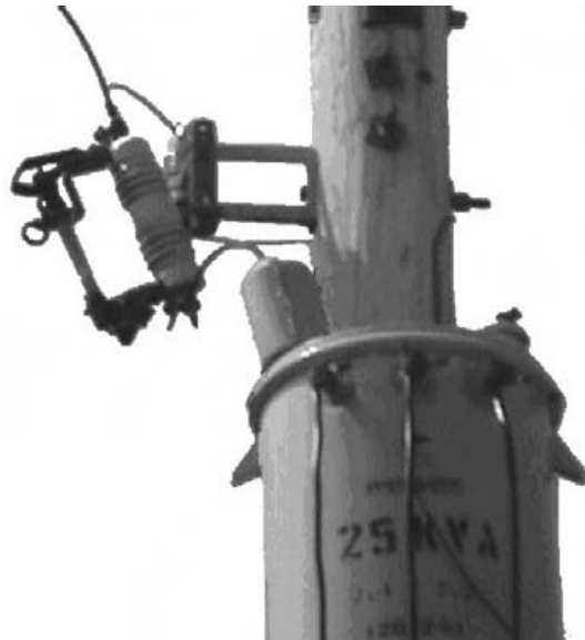
Figure 5.24. Distribution fuses.
