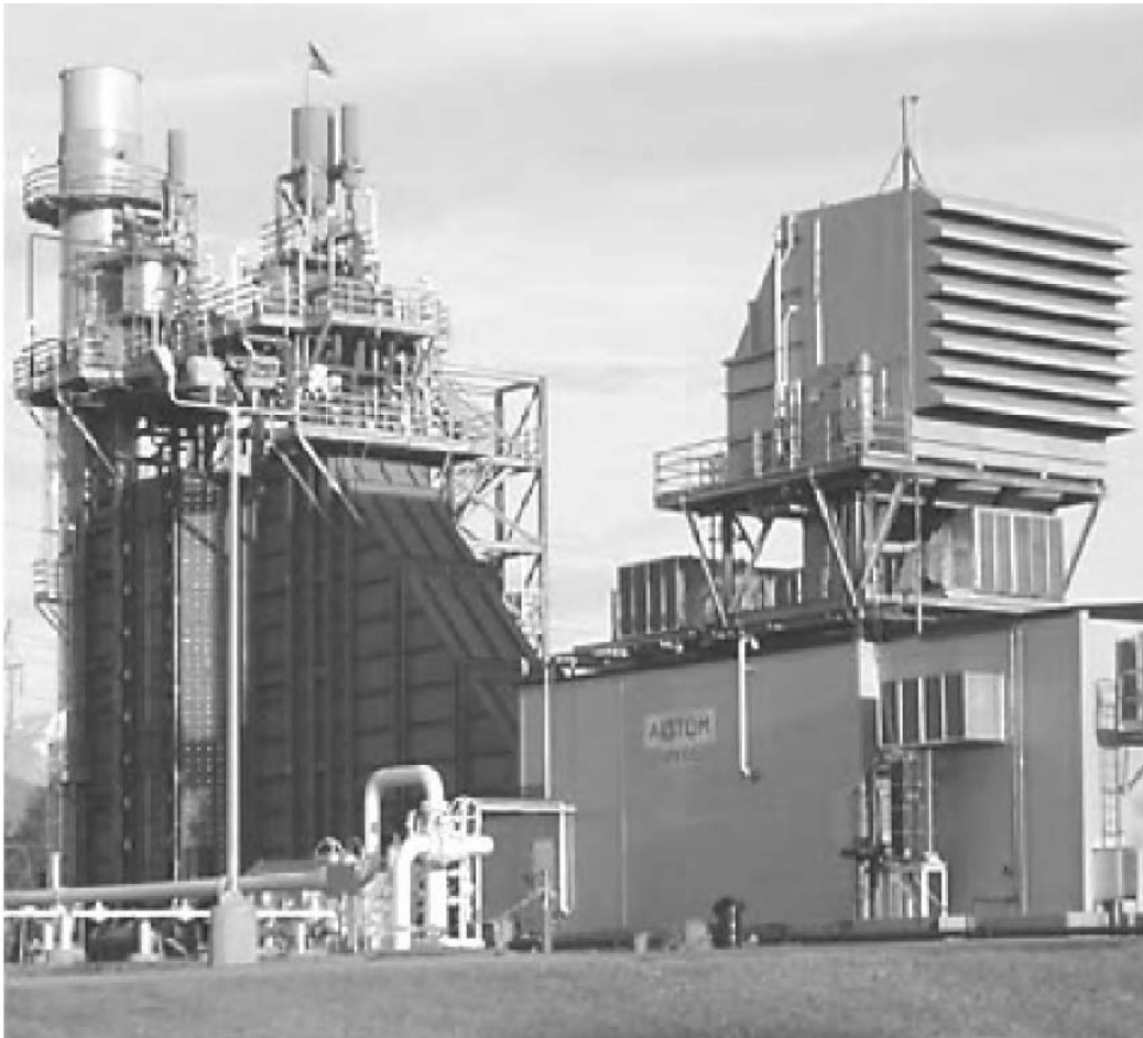
Figure 2-20. Combustion turbine power plant.
