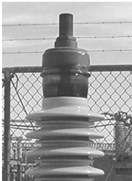
Figure 4-7. Bushing oil level gauge.
